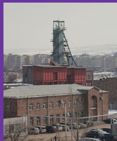
Avan Salt Plant Credit: Amos Chapple
